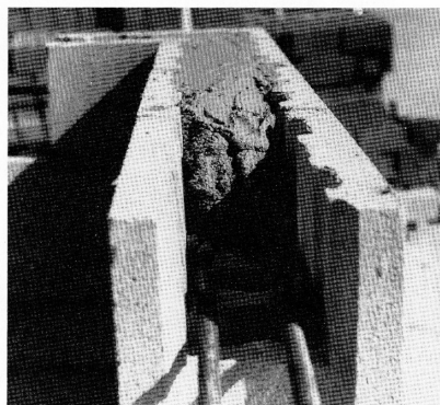
Fig. 6-54. Horizontal reinforcing bars positioned in a bond beam that will be solidly grouted.
