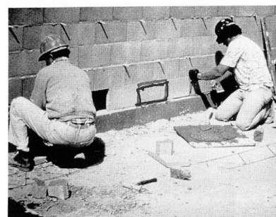
(b) Face Shells Replaced (Usually Only for Exposed Faces)
