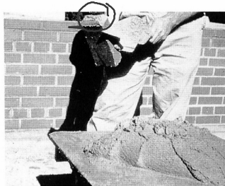
(b) Buttering End of Brick to Ensure Full Head Joints
