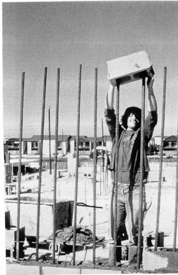
(a) Difficult Placement of Standard Stretchers After the Reinforcement is in Place
