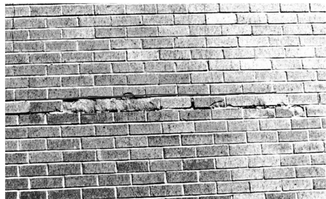
Spalling of brick veneer at shelf angle.
