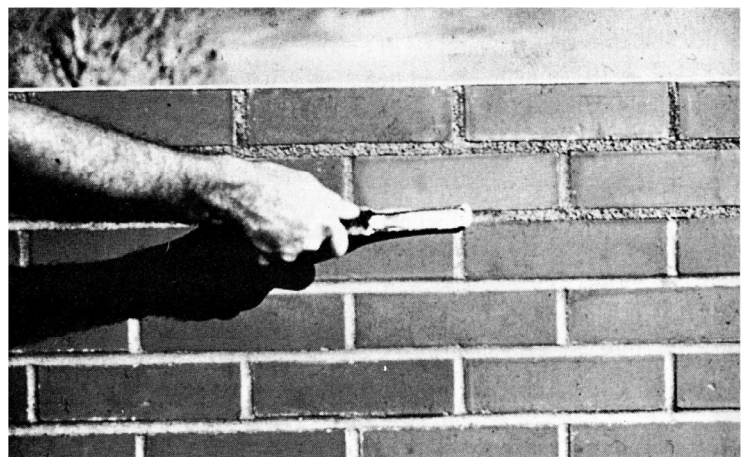
Tooling of mortar joints (concave type)
