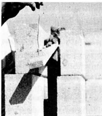
a) Wood strip to remove mortar droppings
