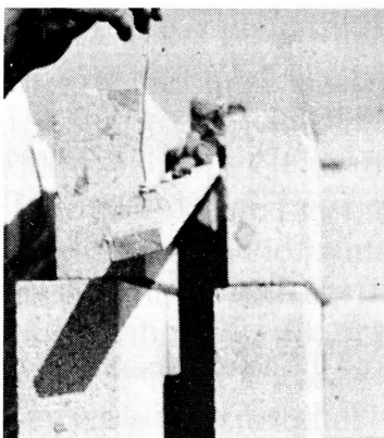
a) Wood strip to remove mortar droppings
