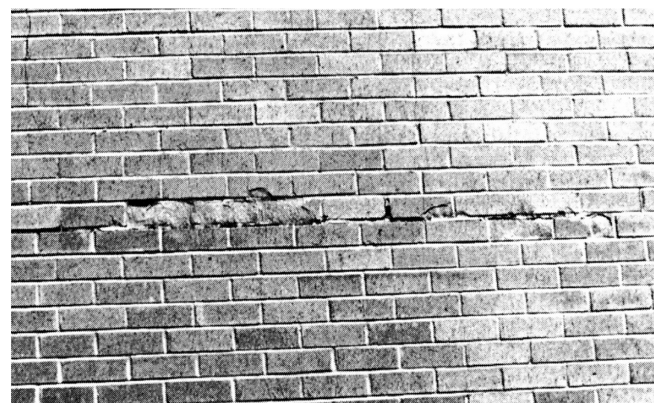
Spalling of brick veneer at shelf angle.
