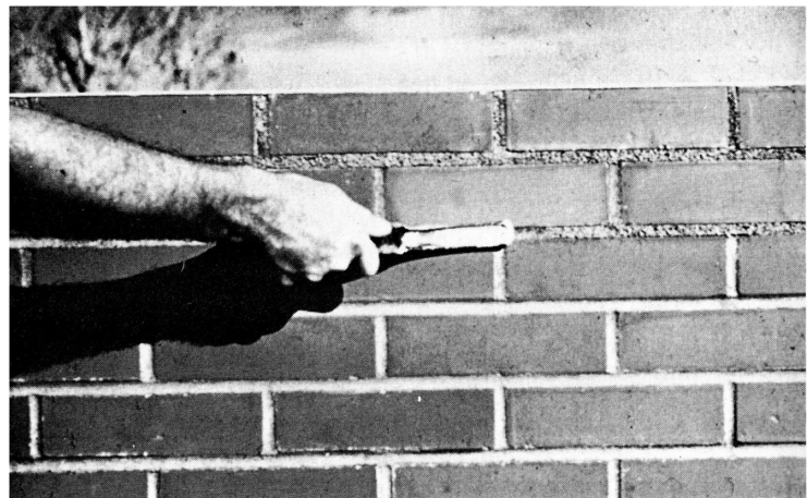
Tooling of mortar joints (concave type)
