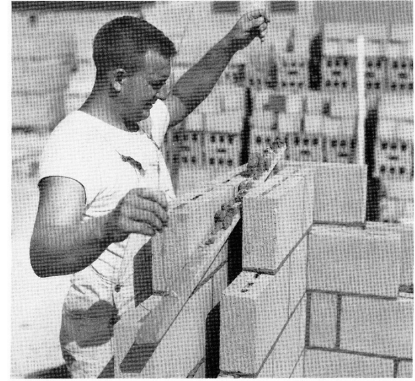
Fig. 6-48. The wood strip is lifted to remove mortar droppings.
