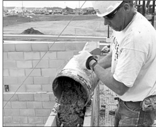
Fig. 6-60. Grouting is stopped about 1 in. below the top of the block to form a key with the next lift.
