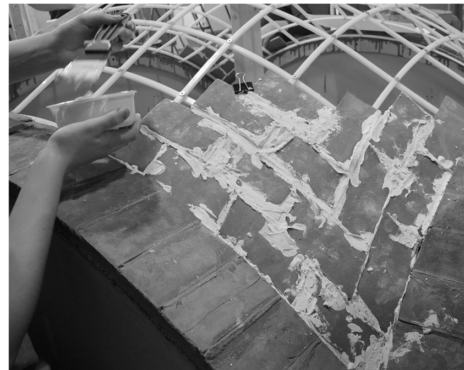
Figure 3: The tiles were placed using mortar and plaster
