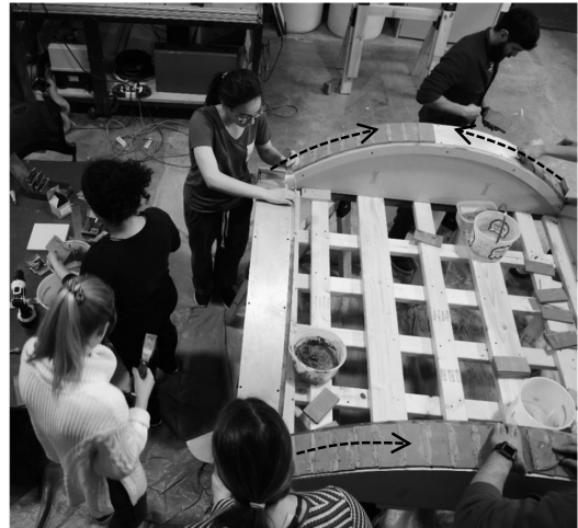
Laying the tiles; red arrows show direction of placement progression
