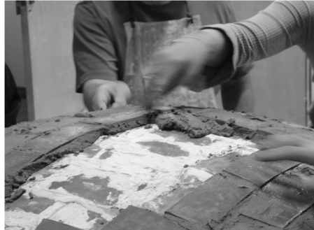
Laying of the mortar bed
