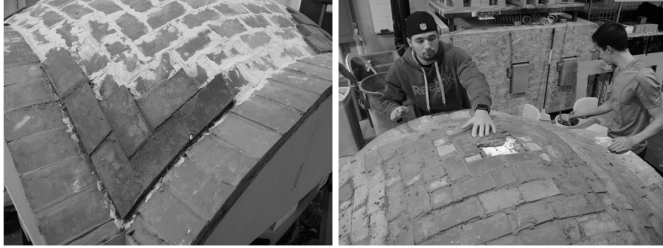
Overlapping pattern of tile layers lent to maximum strength of final design
