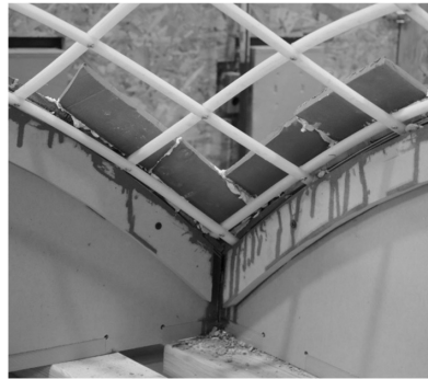
Underside of the grid shell guide at a corner
